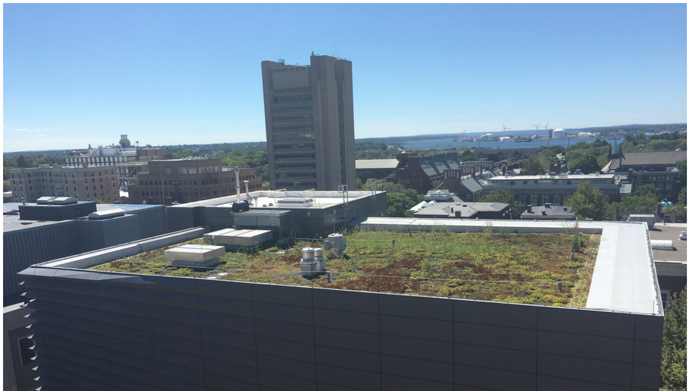
Above: Green roof on top of the Granoff Center
