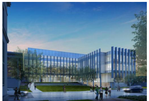
Above: Future view of the school of Engineering Architect: Kieran Timberlake Contractor: Shawmut Design and Construction Scheduled Project Completion: January 2018
