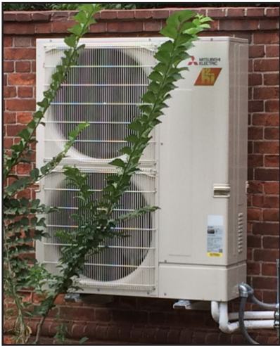
Left: VRF condenser installed at Andrews House. Right: High performance magnetic-bearing chiller installed at Graduate Center
