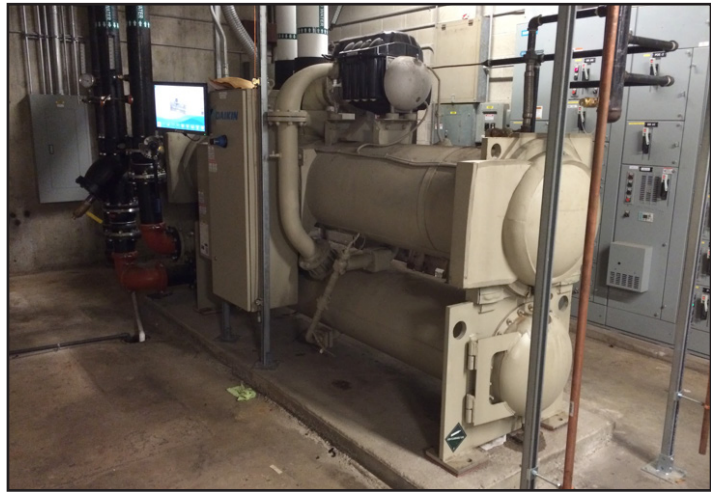
Left: VRF condenser installed at Andrews House. Right: High performance magnetic-bearing chiller installed at Graduate Center
